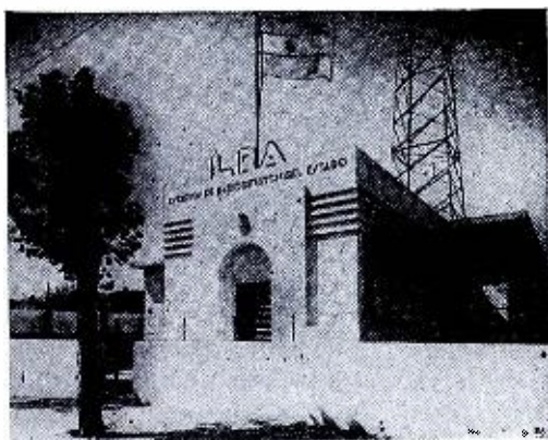
A view of the new building housing the transmitter of Argentine station LRA. This station, known as "Radio del Estado," transmits on 750 kcs with 10,000 watts power.
